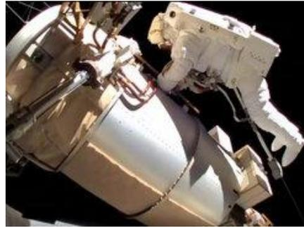
spacewalk replaced a coax feed line installed 11 years ago with another built by the European Space Agency (ESA) and Airbus.
