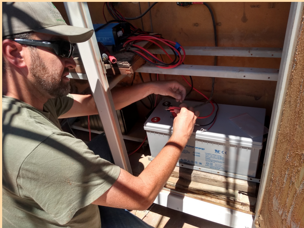
Bryan KF6Y GK connecting new Victron SLA AGM battery. – Photo by Larry AD6G
