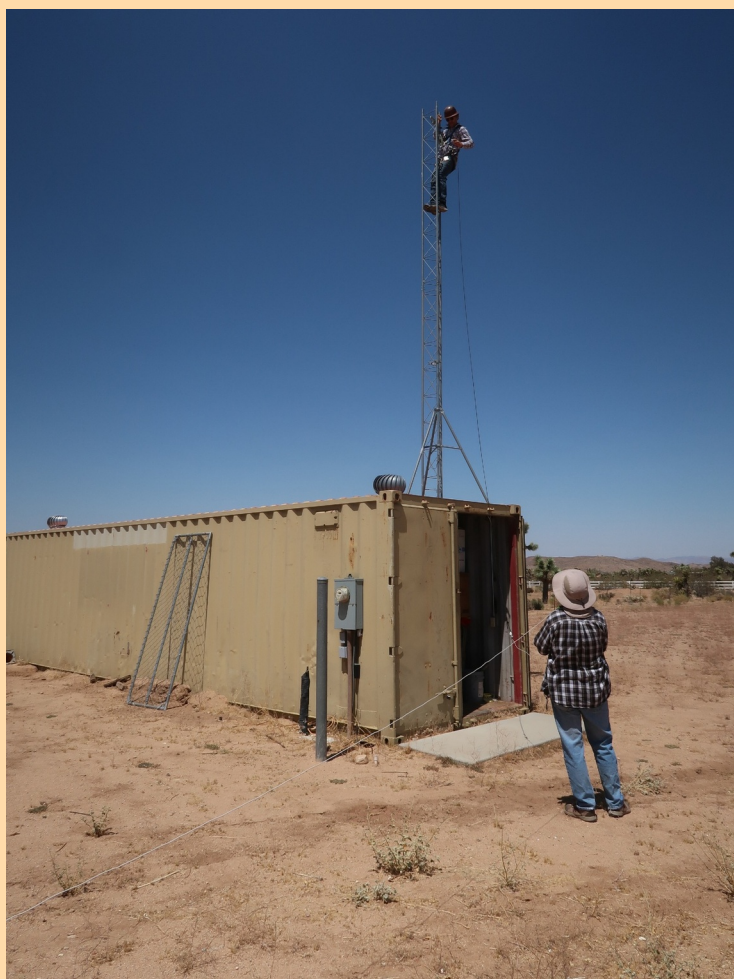
Clifford KK6QMS (on tower) and Larry AD6G prepare to pull up the eastern end of the 80m, 20m, 15m, and 10m end-to-end dipole array. – Photo by Lis Schwitters N6NDC
